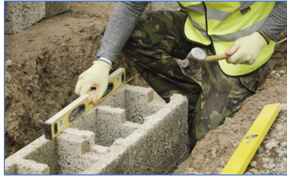
The Durisol unit is bedded onto the mortar and carefully levelled
