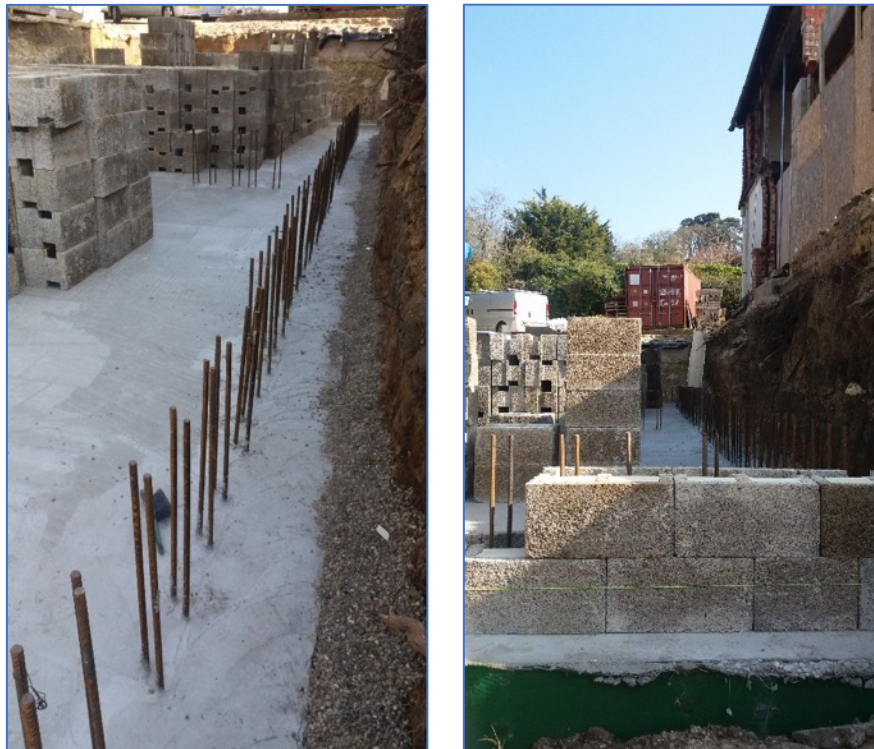
Rebar stubs protruding from a foundation
