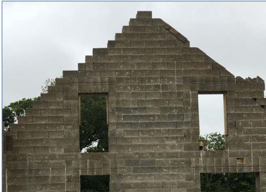
A gable being formed in Durisol units
