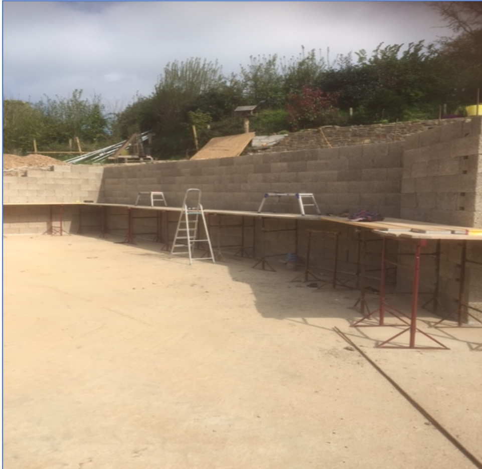
Durisol reinforced concrete retaining wall under construction
