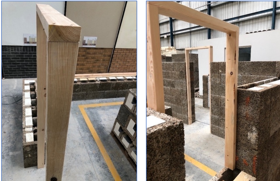
Timber goalposts are used to form openings
