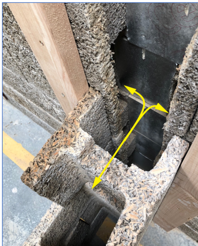
Concrete free to flow at the junction
