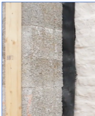
A Durisol wall connected to an existing stone structure
