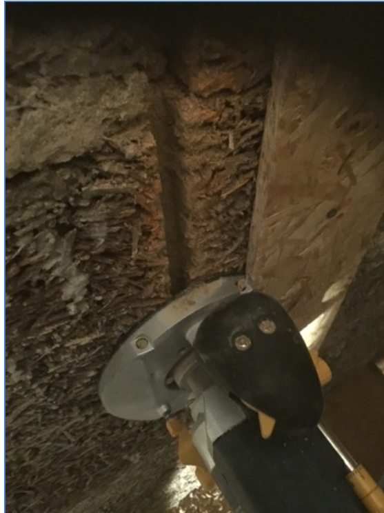
Router being used to chase for services
