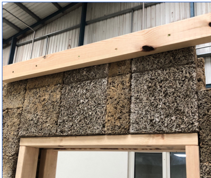
Single door opening braced with 4"x2" secured with coarse threaded 100mm wood screws
