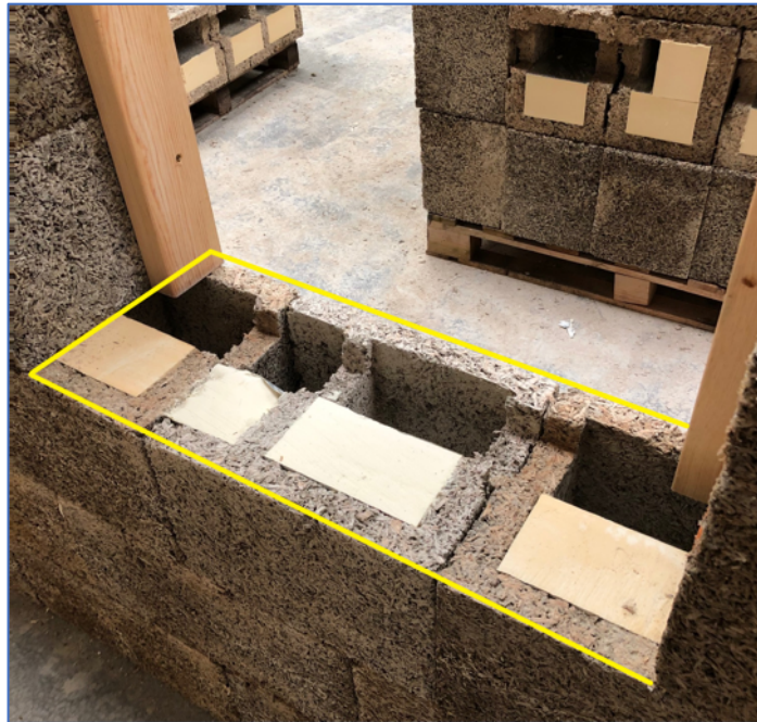
A window opening showing the cill area
