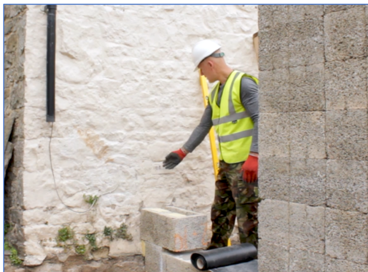
A Durisol wall be constructed perpendicular to an existing wall
