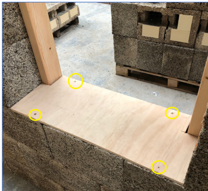
A window cill blanked off with 12-18mm plywood
