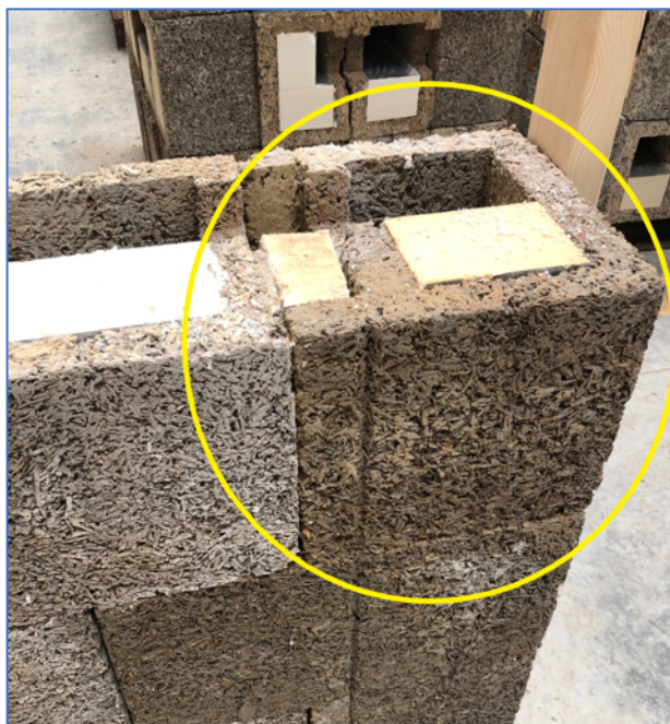
A modified D300 Face Unit inserted into a wall
