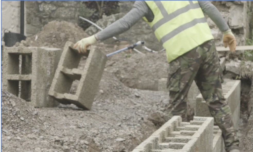
Units should be placed on their ends if they are to stand on the ground before being used
