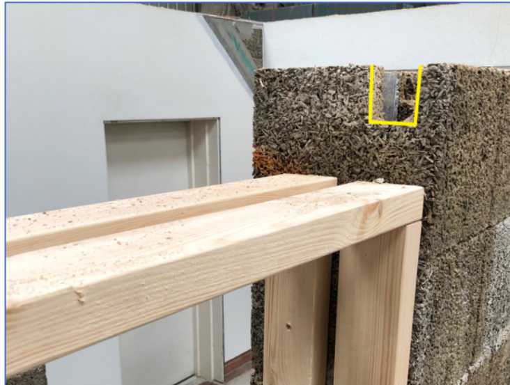
Standard unit adapted to receive reinforcing bars from the end of the lintel
