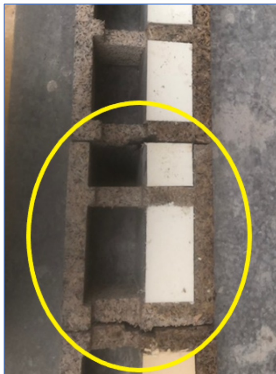
The cut unit is placed in the run of the wall
