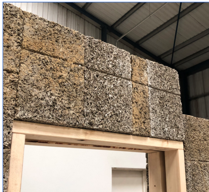
A lintel formed across an opening using face units
