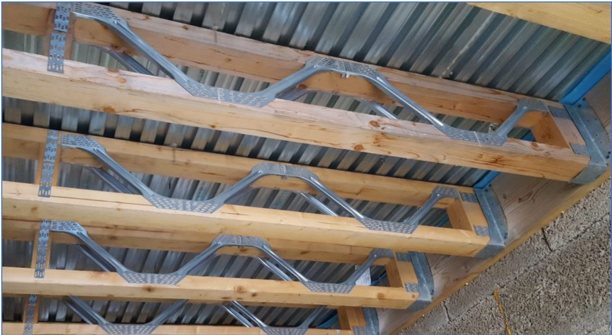
Easi joists supporting a lewis deck floor, spanning onto a timber wall plate bolted to a Durisol wall
