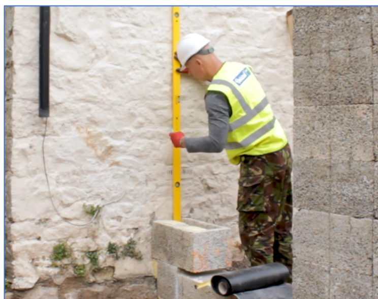
The existing wall should be marked vertically
