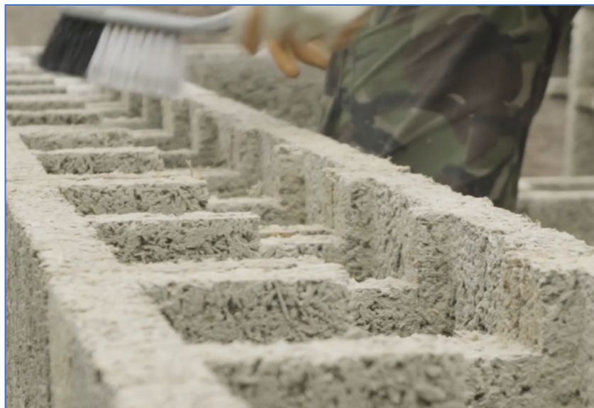
The working top edge of the wall is brushed down between laying courses
