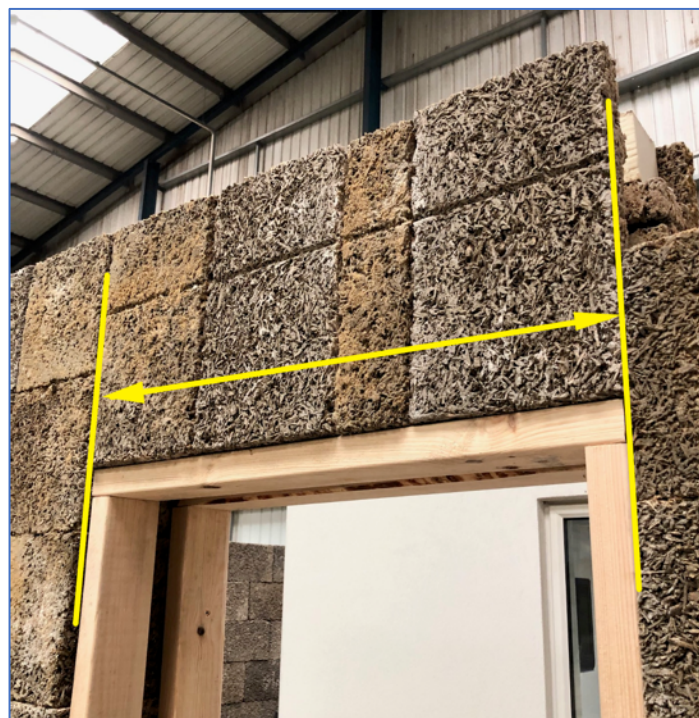
Face units finishing flush with the sides of the opening
