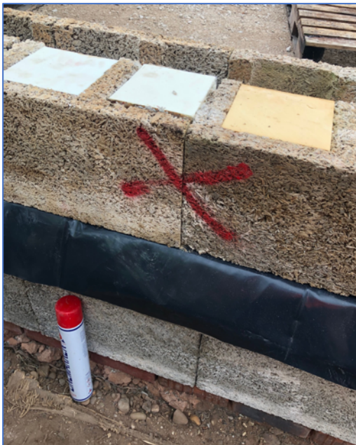
Cut Units being sprayed during placement to mark them for bracing later
