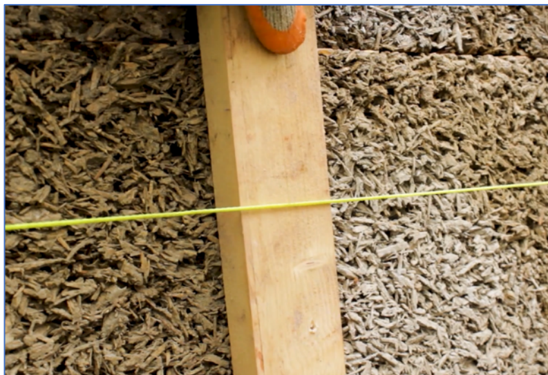
Distance of the string line from the wall can be checked
