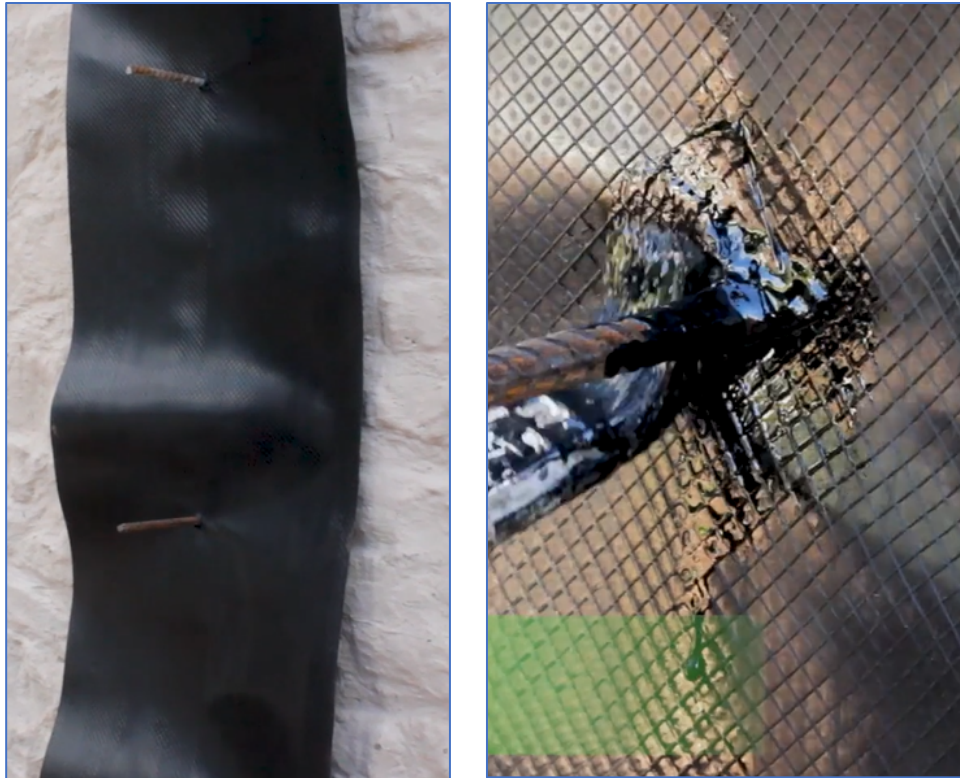
A vertical damp proof course (DPC) is installed and the rebar protrusions are sealed
