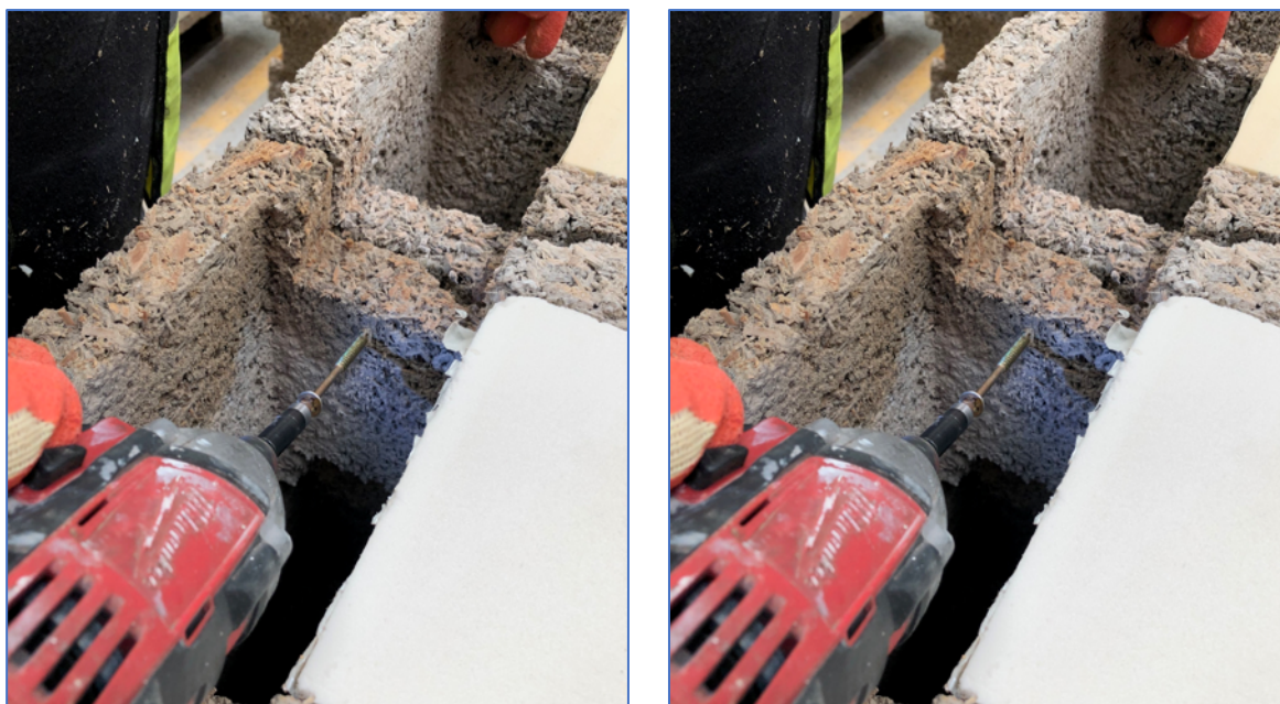
The top course of units can be screwed together with 100mm woodscrews
