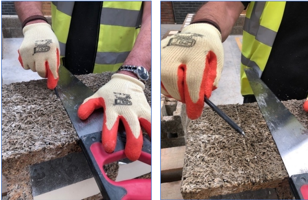
The side of a unit being marked with a tile scorer
