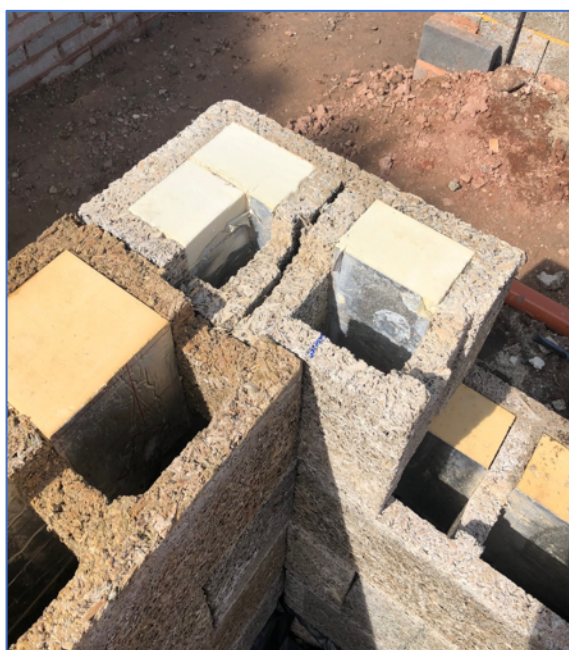
A D365 and D300 wall coming together at a corner
