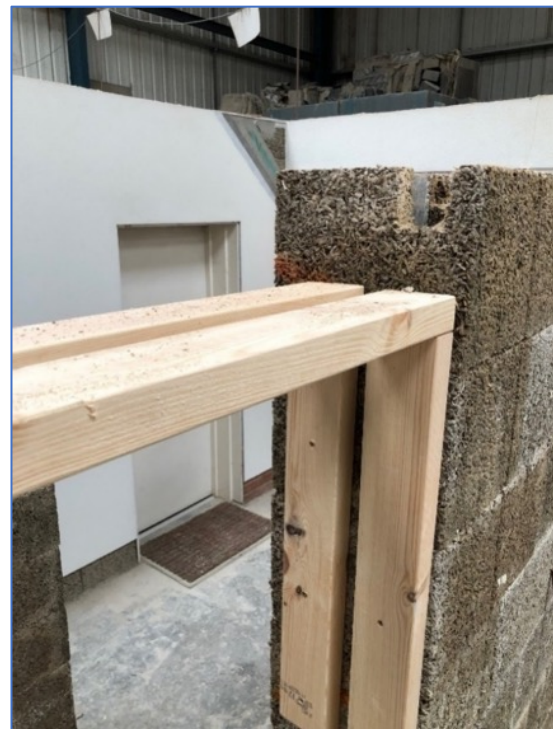
The partial goalpost sits towards the outer face of the wall in line with the insulation inside the units. The vertical uprights of the goalpost are 750mm long and are screwed into the top three courses of units.
