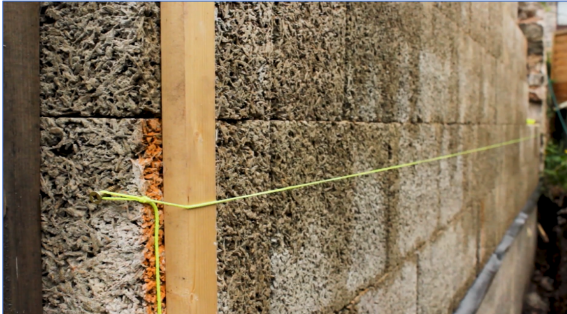
Rig up a string line and use a piece of timber either end to sit it proud of the wall
