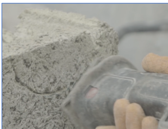
A Durisol unit being cut in a curved shape (with a recip saw) to install pipework
