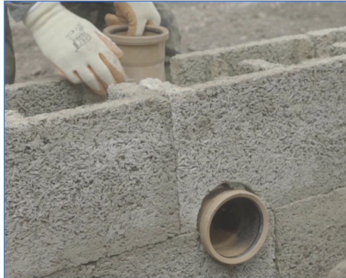
Durisol units shaped to accommodate a waste pipe
