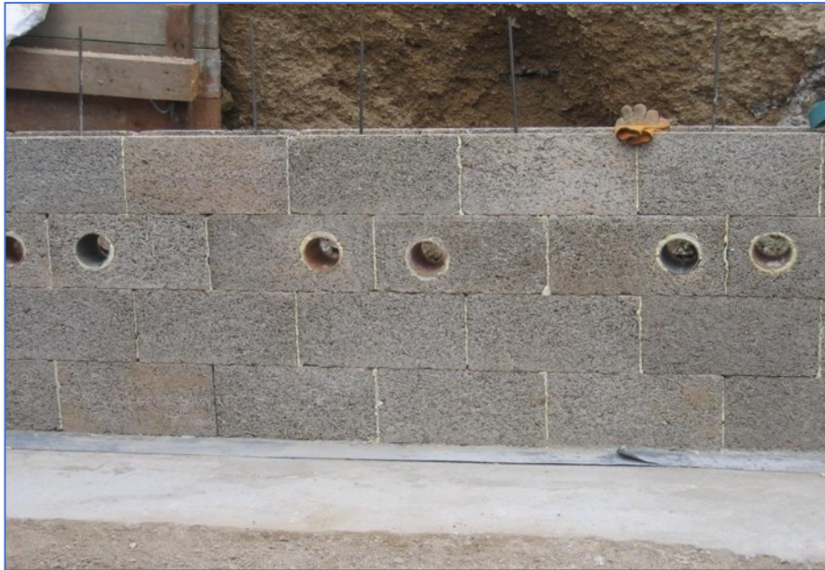
Drainage penetrations formed in a Durisol retaining wall
