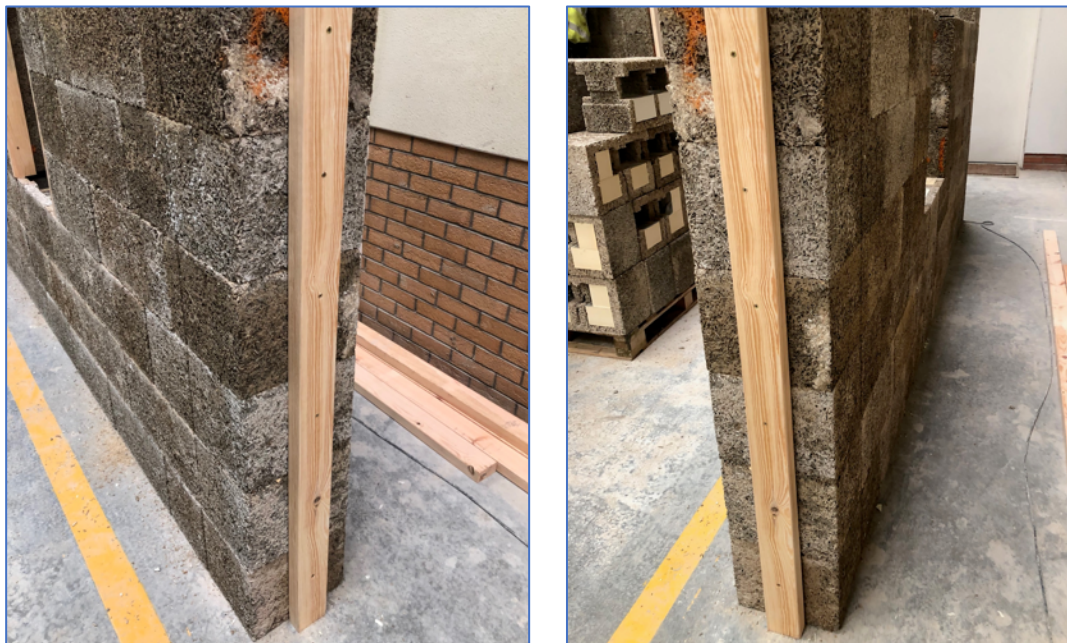
A terminating wall braced with 4"x2" screwed into every unit with a 100mm screw
