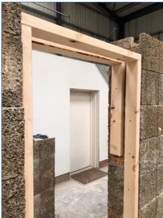
The partial goalpost sits towards the outer face of the wall in line with the insulation inside the units. The vertical uprights of the goalpost are 750mm long and are screwed into the top three courses of units.
