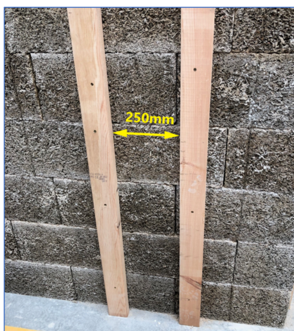
Timber is screwed to the inner face of an external wall to receive a 250mm party wall
