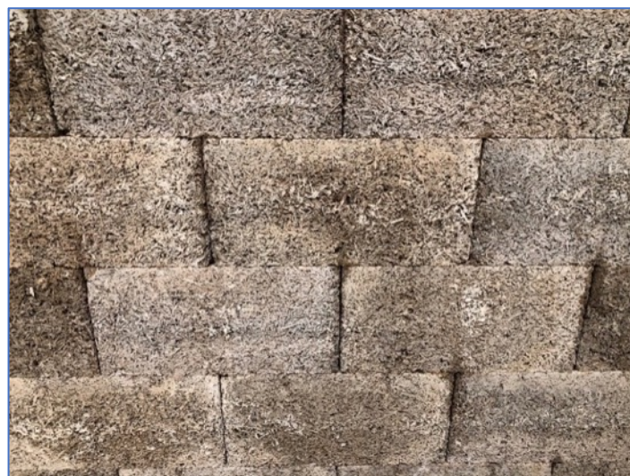
Units stacked in a “brick bond” pattern
