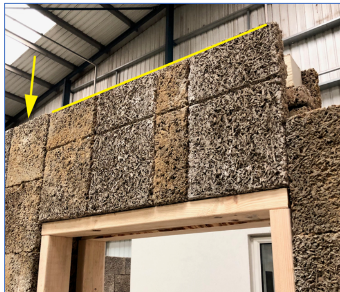
Face units forming lintel cut to bring them back onto course
