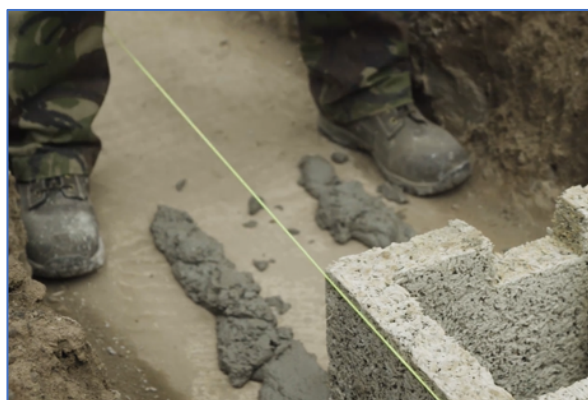
The area is brushed down and a prepared mortar is applied by trowel in two lines
