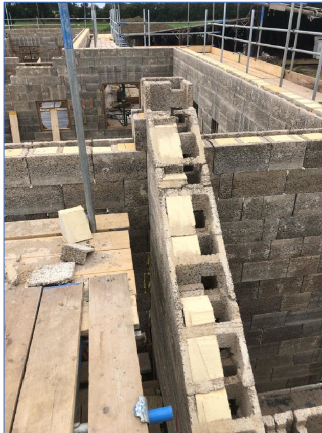
The open top edge of the gable needs to be blanked off with timber before pouring concrete
