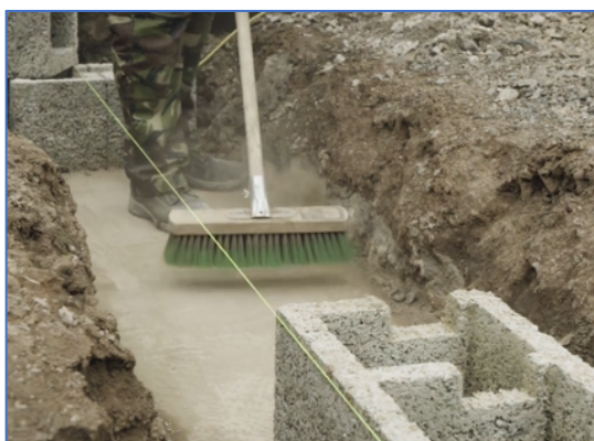
The area is brushed down and a prepared mortar is applied by trowel in two lines
