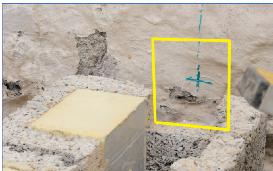
Existing wall marked for installation of rebar stubs
