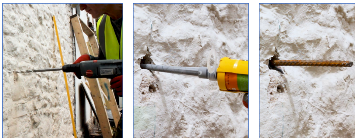
The wall is drilled and a suitable reinforcing bar is resined in to position
