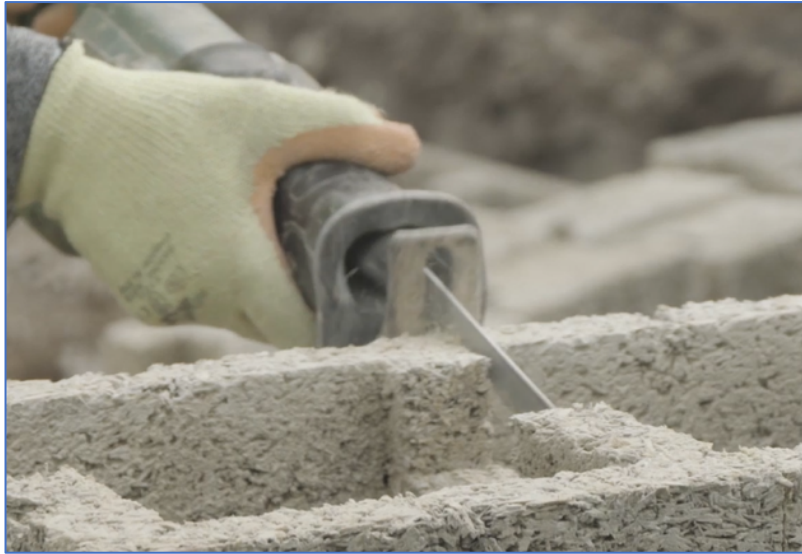
A unit being cut with a reciprocating (recip) saw
