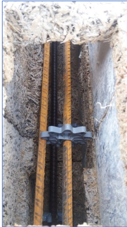
Indicative Rebar on spacers to ensure full encapsulation in the concrete pour
