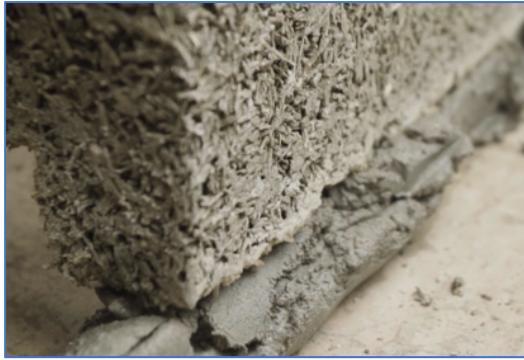
The Durisol unit is bedded onto the mortar and carefully levelled
