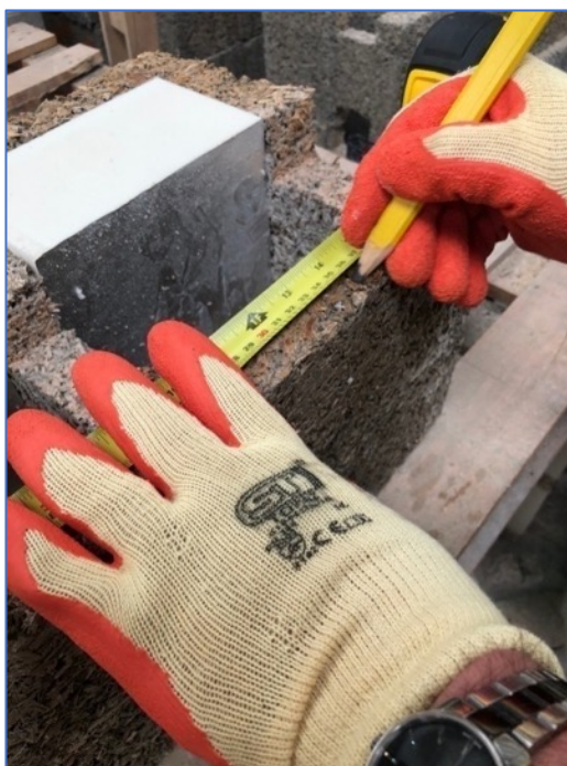
The top of a unit being marked with a pencil
