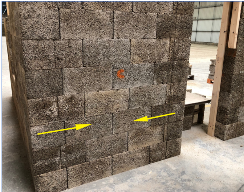
Build from the corners and openings towards the midspans
