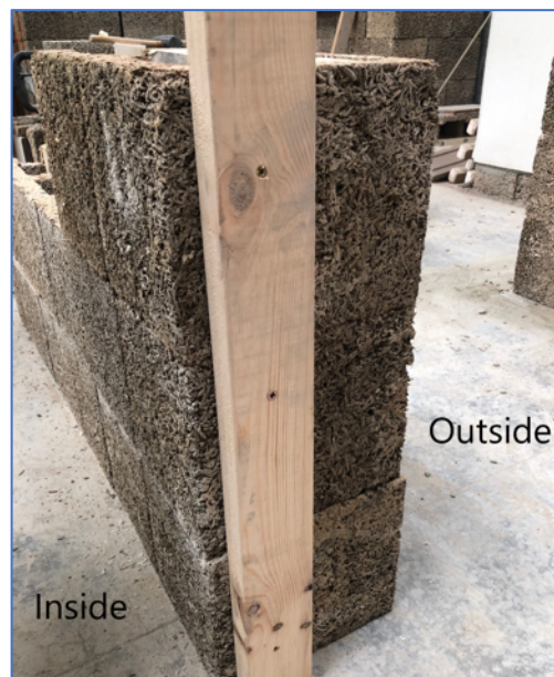
The full height timber goalpost for a door opening
