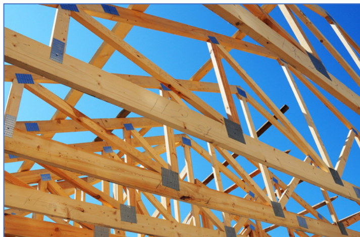
Closed timber roof trusses with horizontal tie beams
