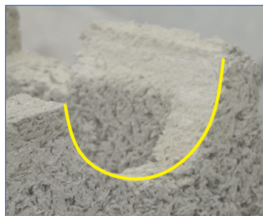
A Durisol unit being cut in a curved shape (with a recip saw) to install pipework
