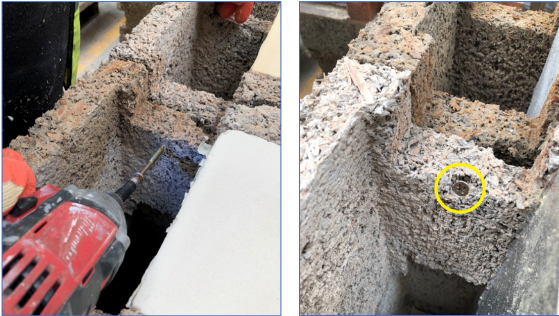
The top course of units can be screwed together with 100mm woodscrews
