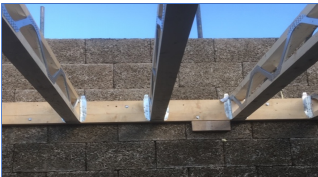
Posi joists sitting in joist hangers and bolted to the core of a Durisol wall via a timber wall plate
