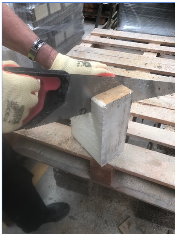
Insulation being cut with a handsaw
