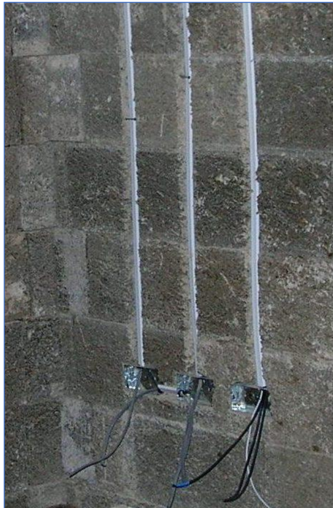
First fix electrical wiring and conduit being installed
