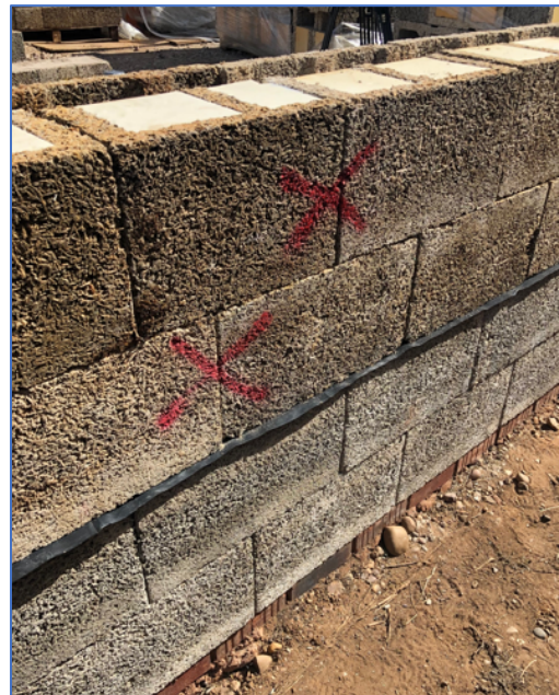
Cut Units being sprayed during placement to mark them for bracing later
