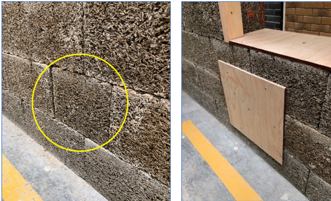
A cut unit in a wall being braced with ply
