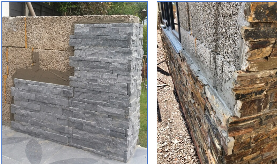
Indicative stone slip cladding bonded directly to Durisol units
