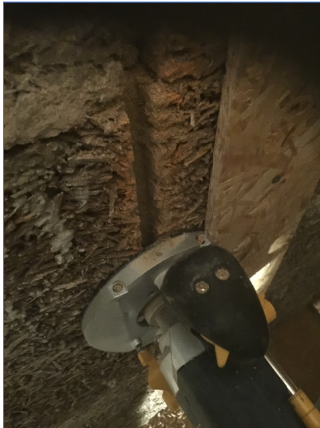
A router being used to create recesses
