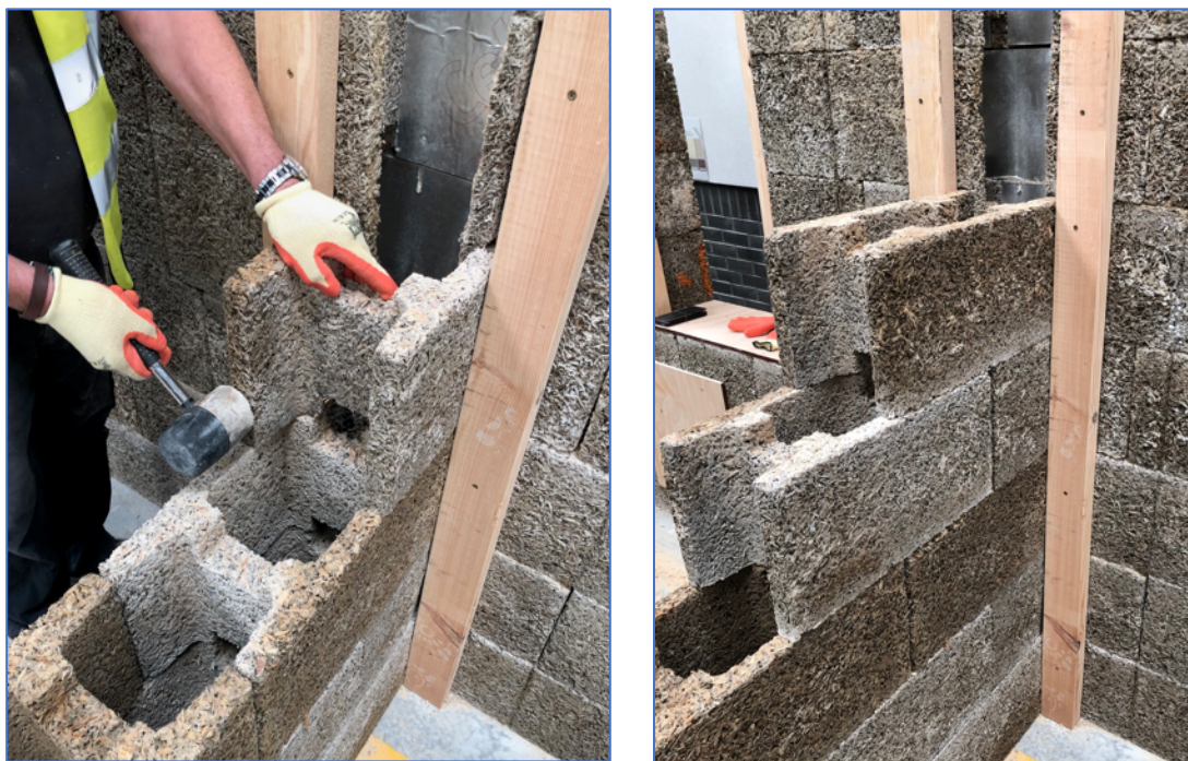
A D250 party wall being built against a prepared external wall
