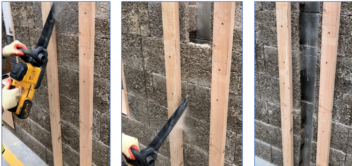
A 180mm wide channel is cut out of the external wall (inner leaf) to join a D250 party wall.
