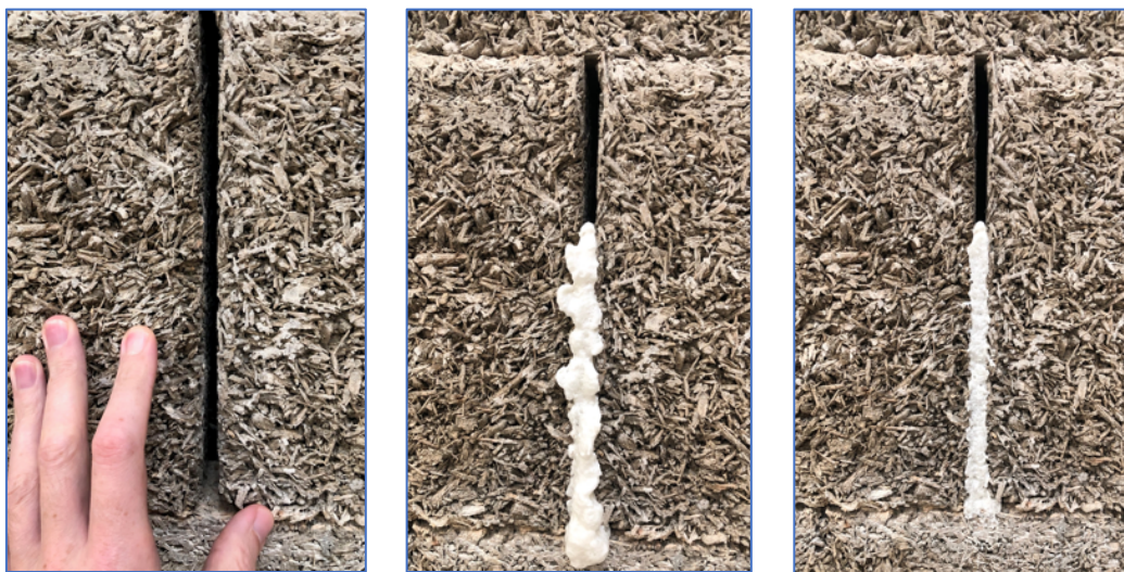
A vertical gap between units being filled with fire rated foam and then cut off flush once dry (in practice the gap would be filled completely from top to bottom)
